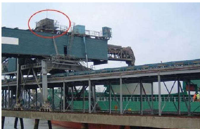
Grain conveyor transfer point with fog
