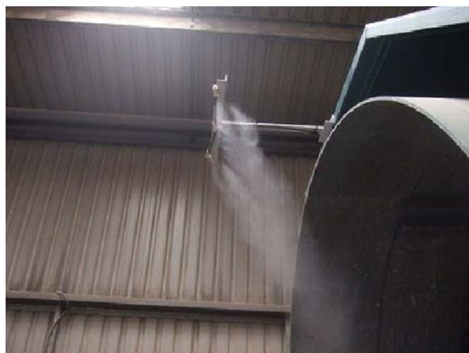
Fog protecting a trommel outfeed
