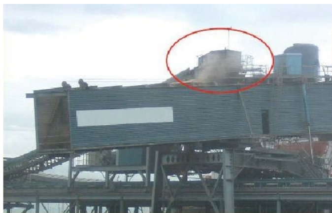
Grain conveyor transfer point without fog
