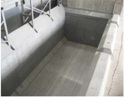
Oslo / Norway Waste recycling
