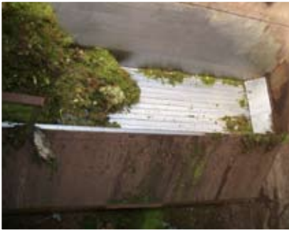
Luxemburg Composting Factory
